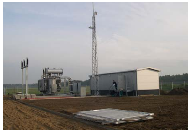
Substation construction at the Site
