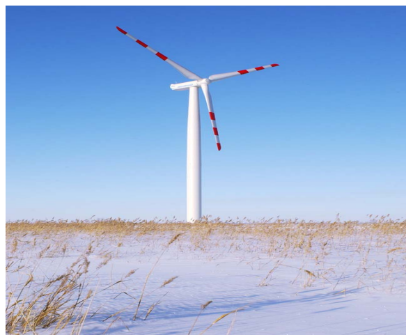
WWD 3 Turbines (Photo from www.winwind.fi )
