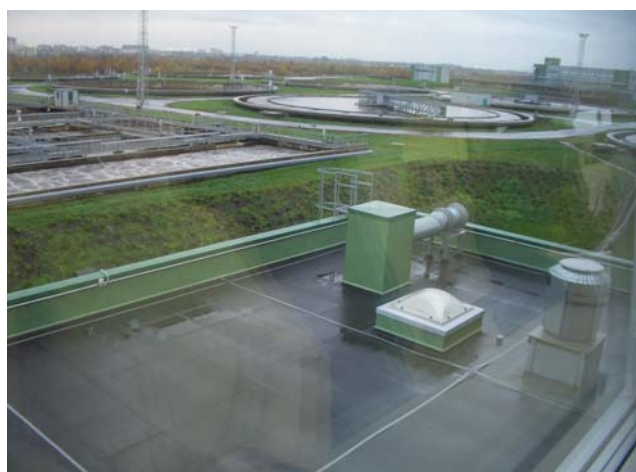
Primary Sedimentation Tanks at South West WWTP
