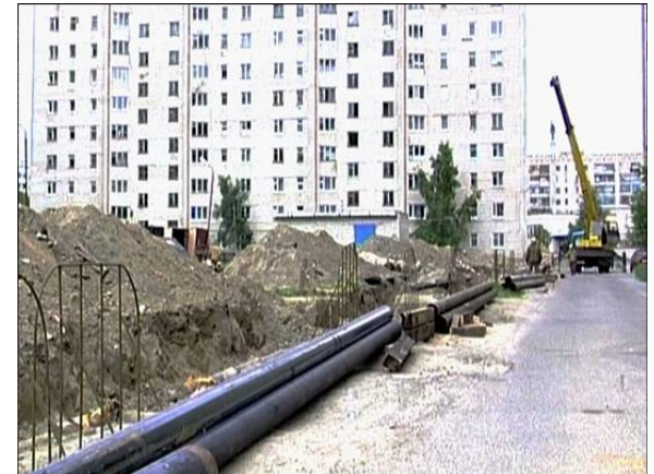
Network Reconstruction Works, Strezhevoi
