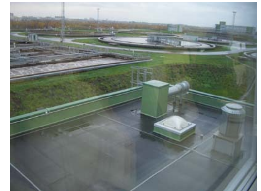
Sedimentation Tanks at SW WWTP
