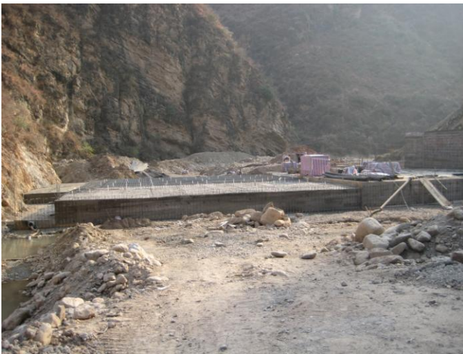
Figure 2 The damn/reservoir construction status as of Feb 2010
