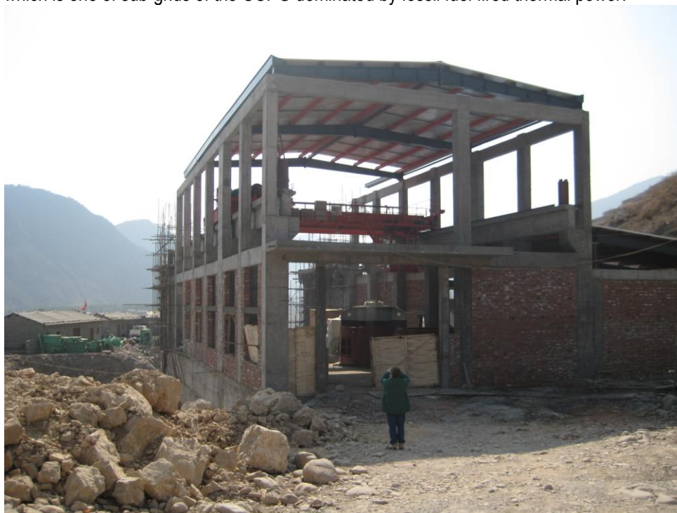
Figure 1 The power house construction status as of Feb 2010.
