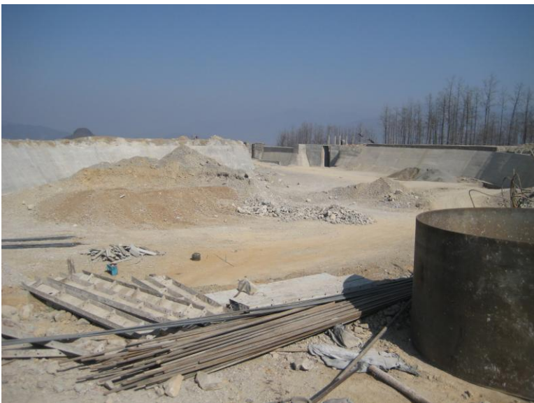
Figure 2 The reservoir construction status as of Feb 2010.
