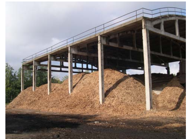
Biomass Resources, Priozersk
