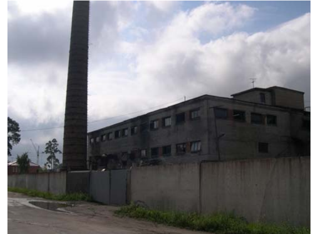
Old Boiler House, Priozersk
