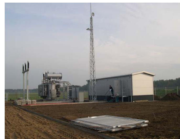
Substation construction in Oct 2006
