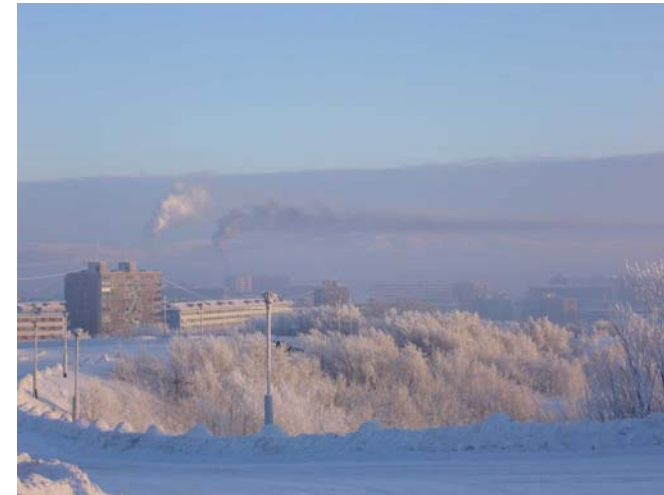
Severnaya Heat Plant
