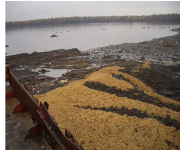
Existing Sludge Lagoon for SW WWTP
