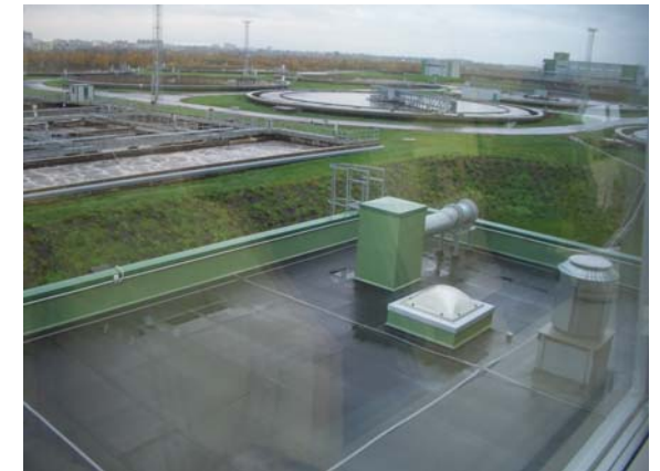
Sedimentation Tanks at SW WWTP
