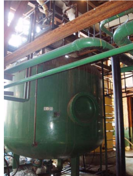
Existing Gas Boilers
