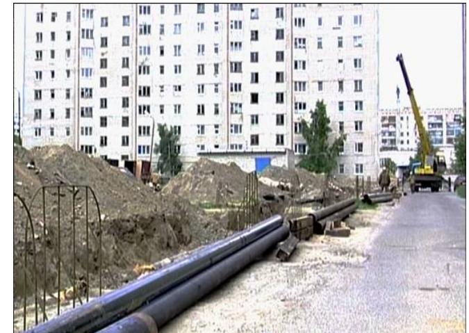
Network Reconstruction Works, Strezhevoi
