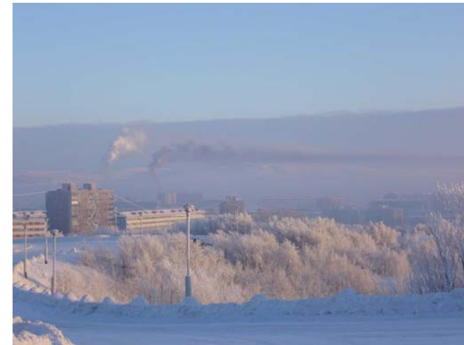
Severnaya Heat Plant
