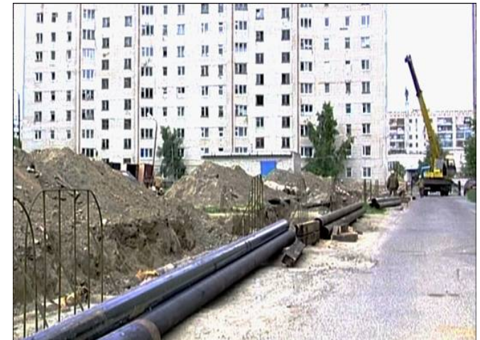
Network Reconstruction Works, Strezhevoi
