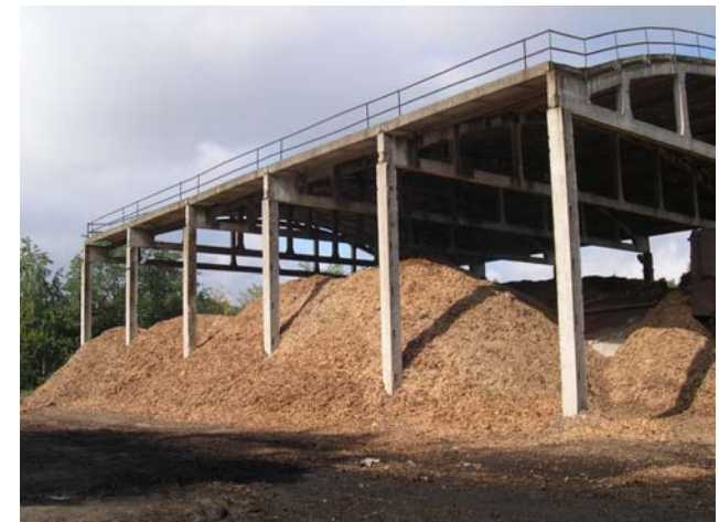
Biomass Resources, Priozersk
