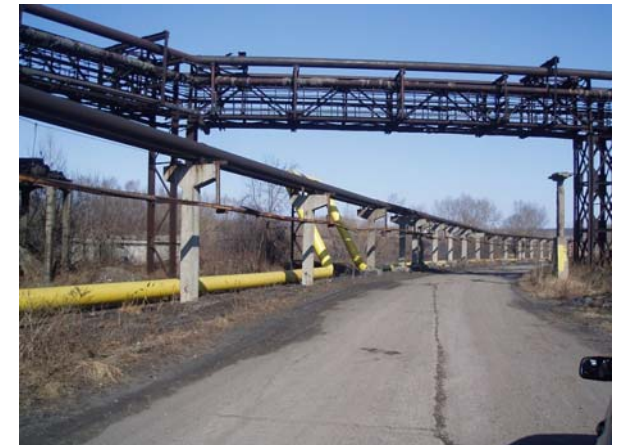
Old Natural Gas Pipeline
