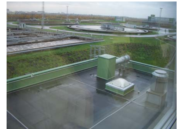
Sedimentation Tanks at SW WWTP
