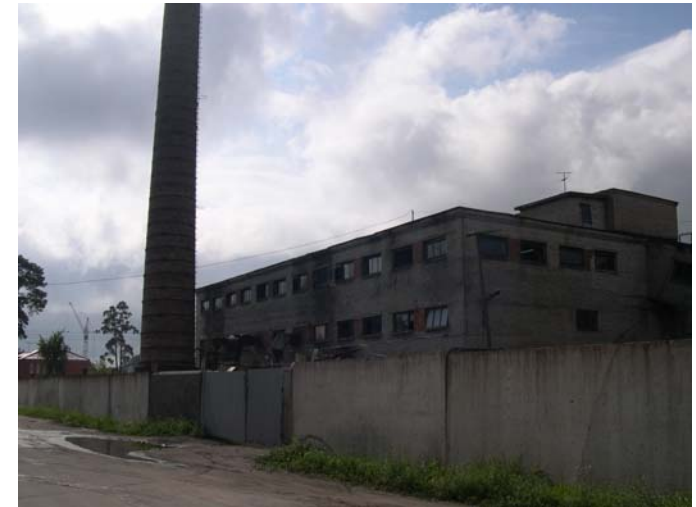
Old Boiler House, Priozersk
