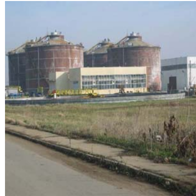
Digestors and Pumping Station for raw sewage, Kubratovo, Sofia
