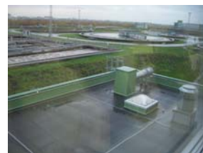
Sedimentation Tanks at SW WWTP
