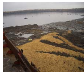
Existing Sludge Lagoon for SW WWTP
