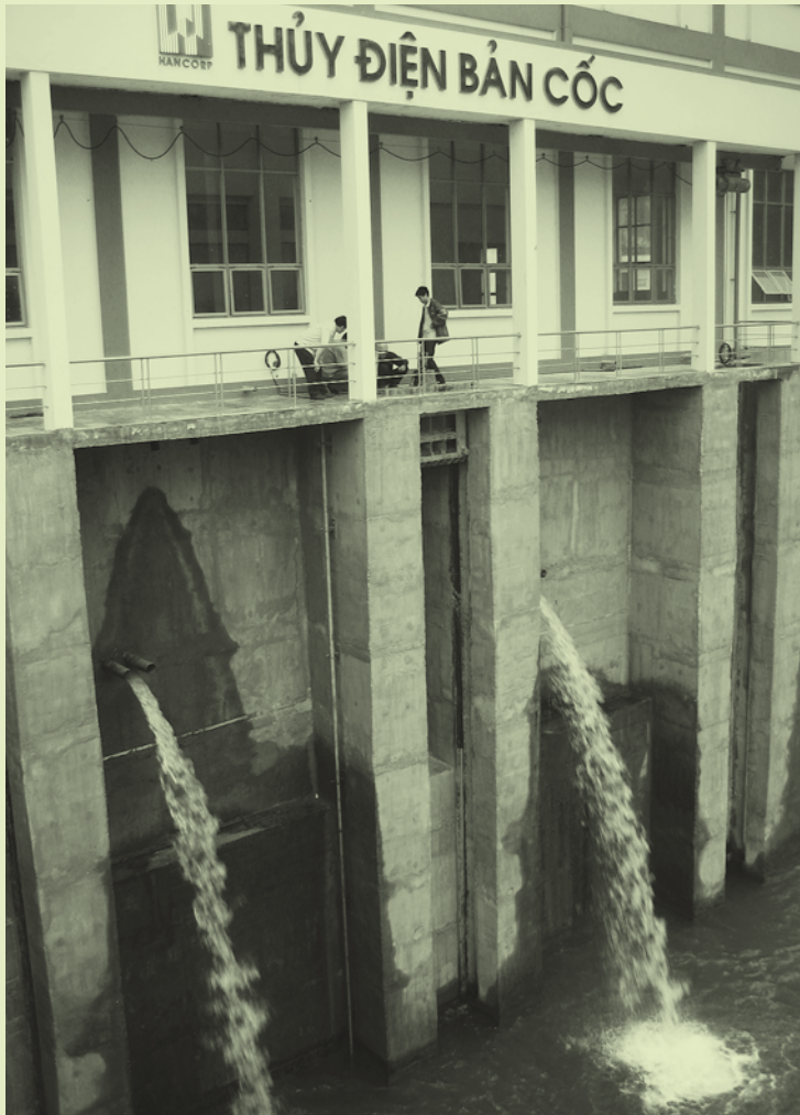
The Ban Coc hydro power-house generates approximately 75 Gwh renewable energy per year. Photo: Maija Saijonmaa
