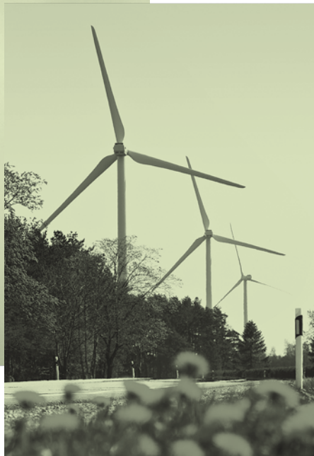
Estonia registered NEFCO's first wind farm project under the national JI-track 1 in December 2009. Photo: Nelja Energia
