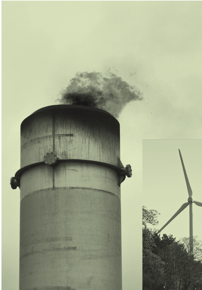
Chimney at Lapes, Lithuania. TGF's Lapes landfill gas utilisation project achieved its final JI-determination in January 2010. Photo: Hanna-Mari Ahonen
