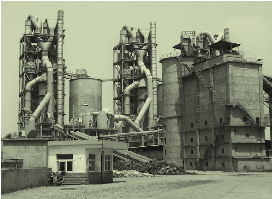
Cement production in the Jiangsu province in China. The project utilises waste heat from the cement production to generate power. Photo: Maija Saijonmaa
