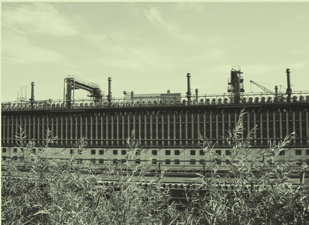
Coke battery at Alchevsk coke plant in Ukraine. Photo: CF Partners
